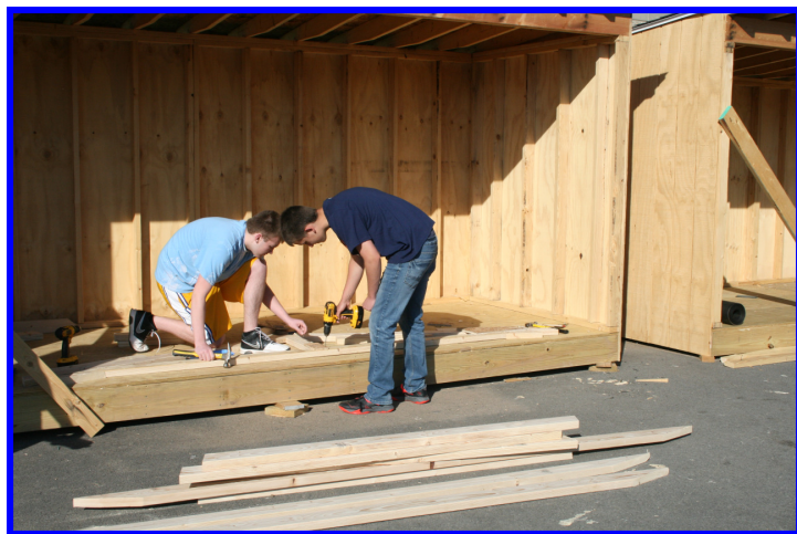
LtoR: Connor McGrath & Ricci Shenck work on a truss in dugout
