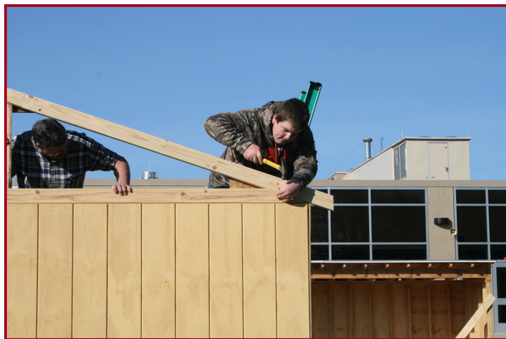
Kyle Ierlan nails a truss to the shed while teacher Tim Rogers supervises.
